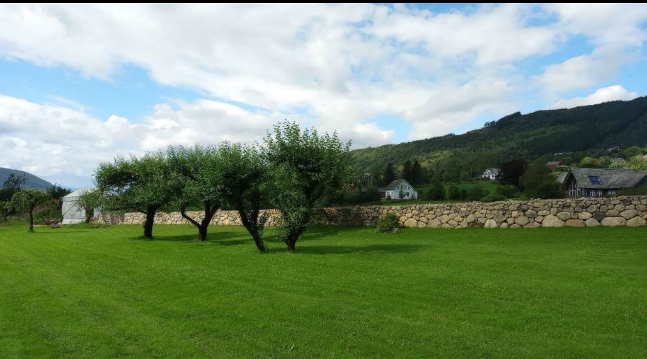
Ongoing restoration projects nearing completion – the kitchen garden wall: before and after
